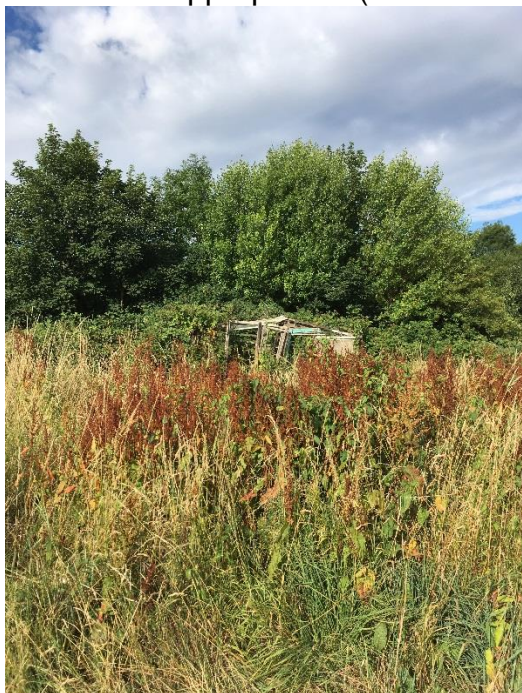
Abandoned plots with derelict structures
